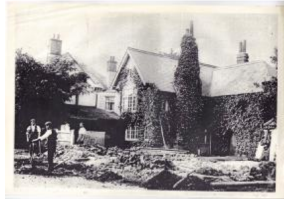
Ash Green House reconstruction in the early 1900s
